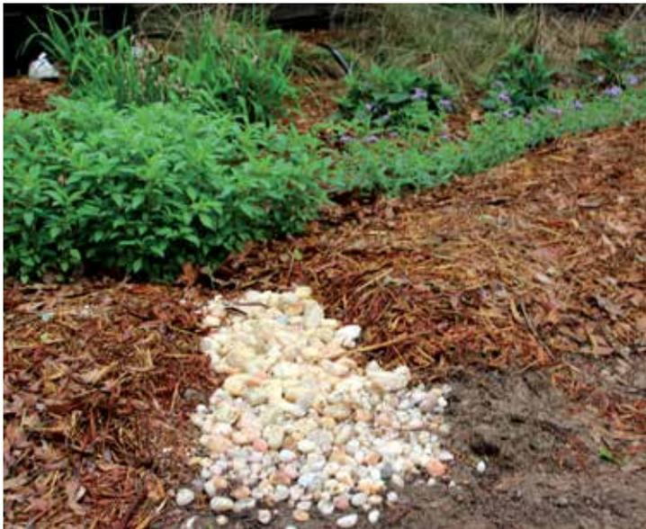
*Rocks can be used to reinforce the berm, allowing for overflow during heavy rainfalls.*
